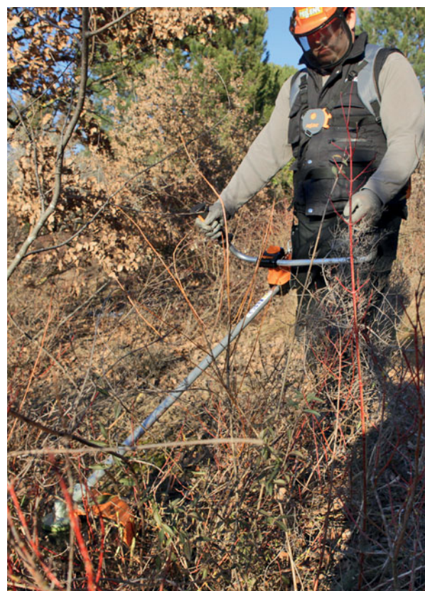
Site clearing in a thicket
