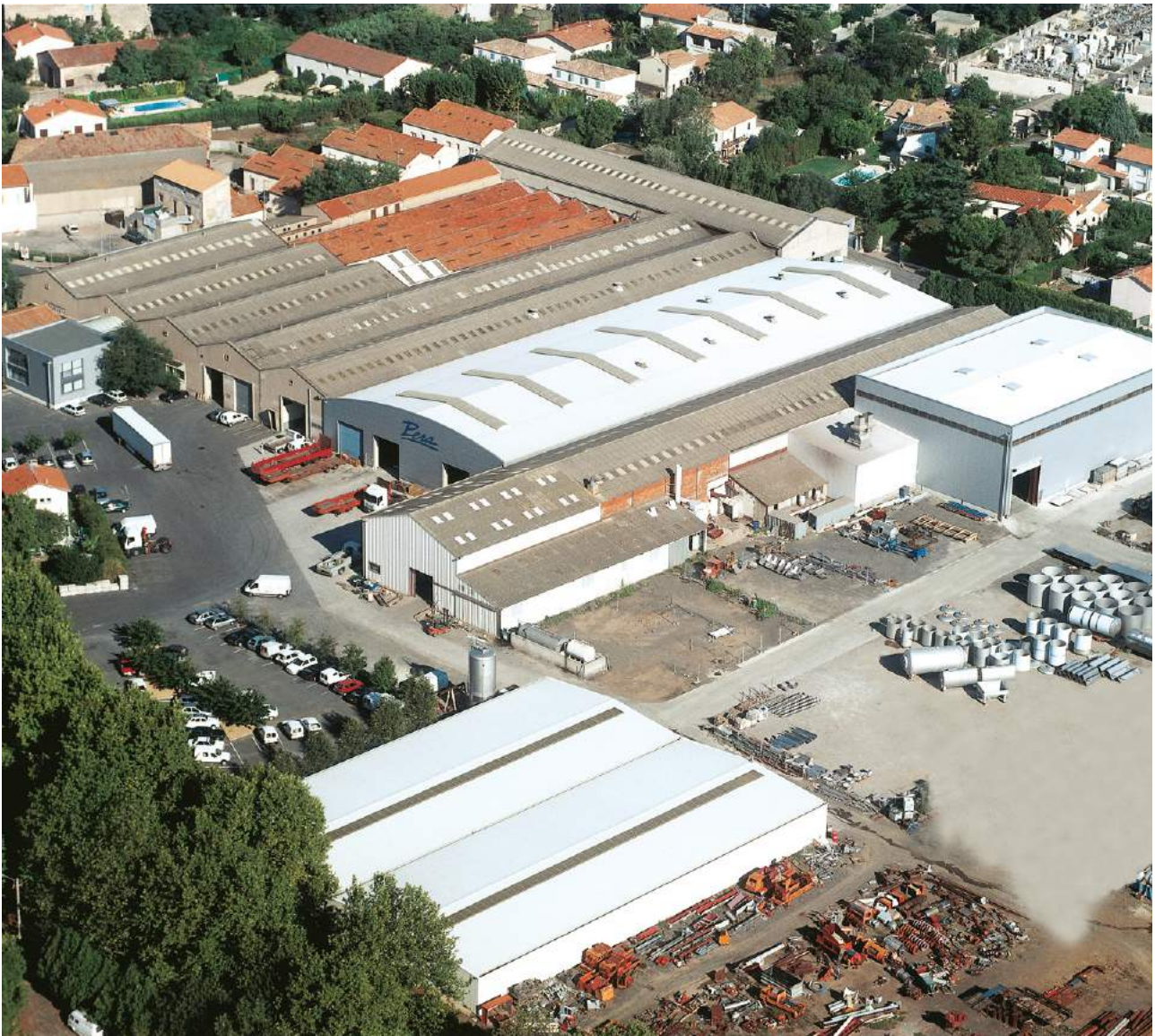
The headquarters of PERA-PELLENC in Florensac (34) - France
